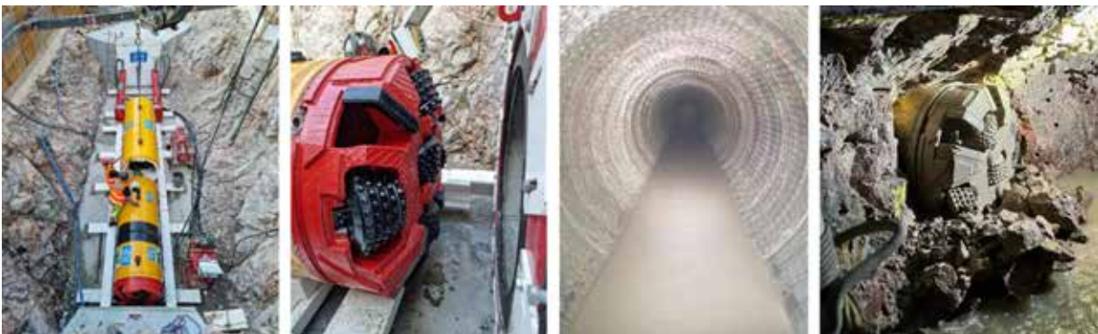
Figure 8. AVN 800 HR (for OD 1110 mm) in operation in Edsberg, Sweden
